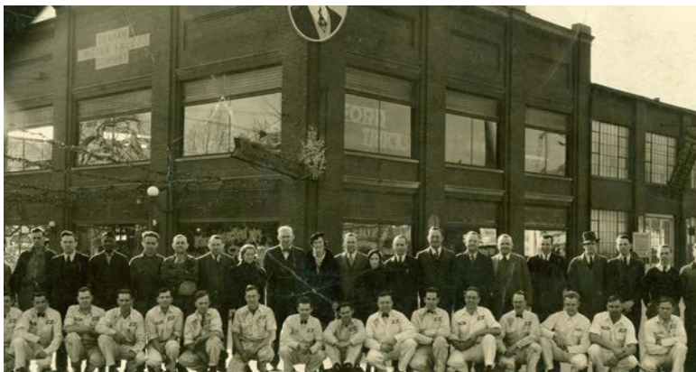
Graham Motor Sales Company Building, Bloomington, Indiana. ca. 1935.
